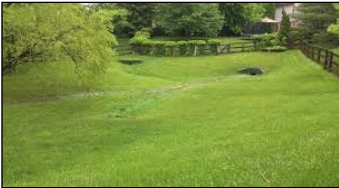
An example of a detention basin.
