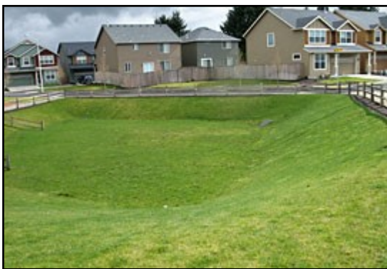
A detention stormwater basin in a neighborhood.
